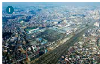
1 MFTBC Headquarters Kawasaki Plant / Research & Development and Purchasing Center Kawasaki City, Kanagawa
